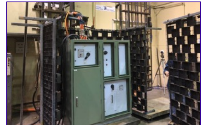
Top: 'Fail test' to identify arc-fault hazard Btm: Certified safe containment – no doors
